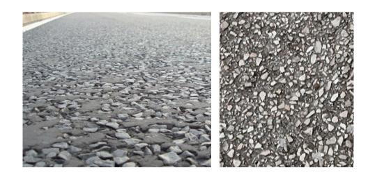
The raised- / shared surface will be finished in hot rolled asphalt with
